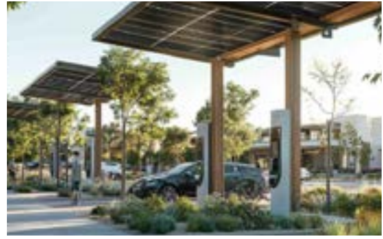
SOLAR CHARGING STATION
